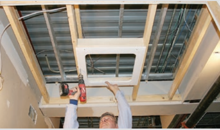
2. Mount Seamless™ surround with drywall with screws
