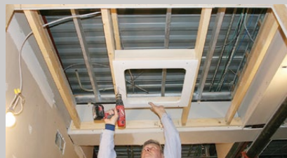
2. Mount Seamless™ surround with drywall with screws
