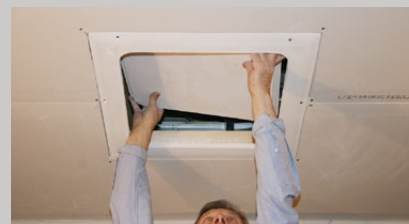
4. Install drywall and place access panel in opening
