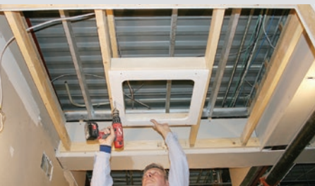
2. Mount Seamless™ surround with drywall with screws
